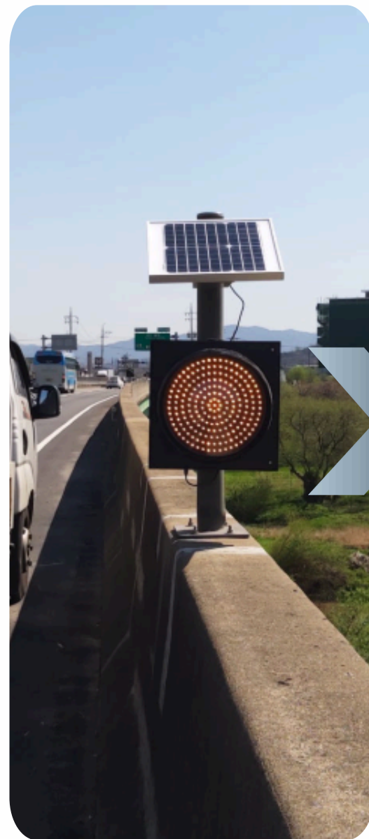
Conventional Solar-Powered System
